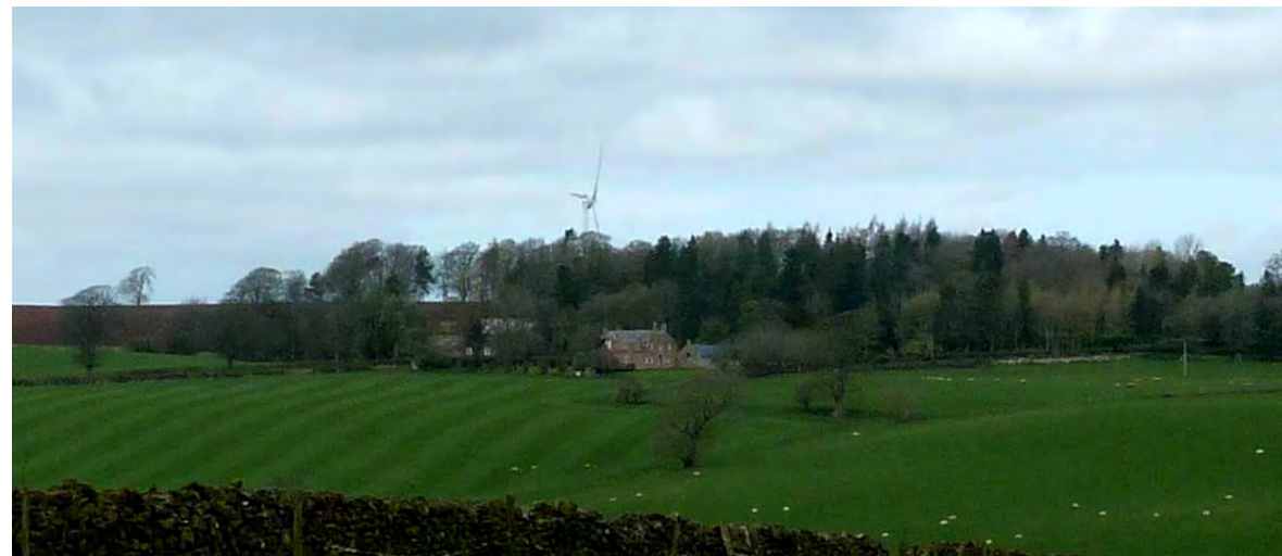
67m turbine at Bassendeanhill in the Westruther Platform LCA. This location was considered unsuitable by SBC, but subsequently granted on appeal
